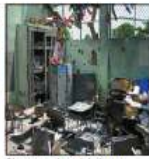
Classroom devastated as a result of aerial bombing by SLAF
